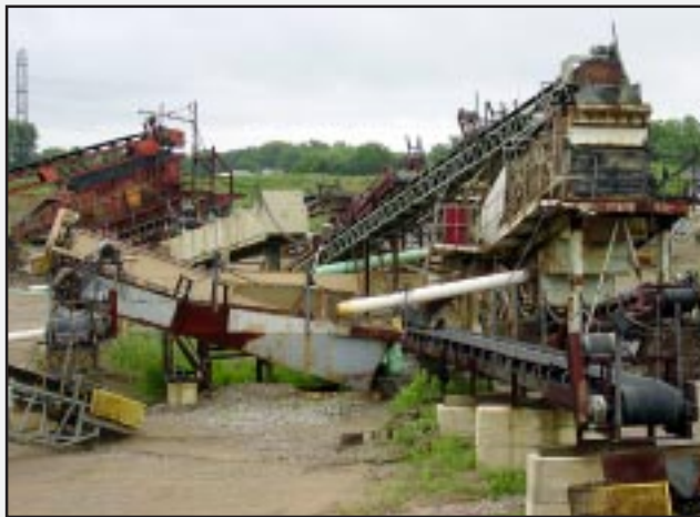
Overview of Plant
